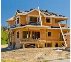
Residential New Home Construction
