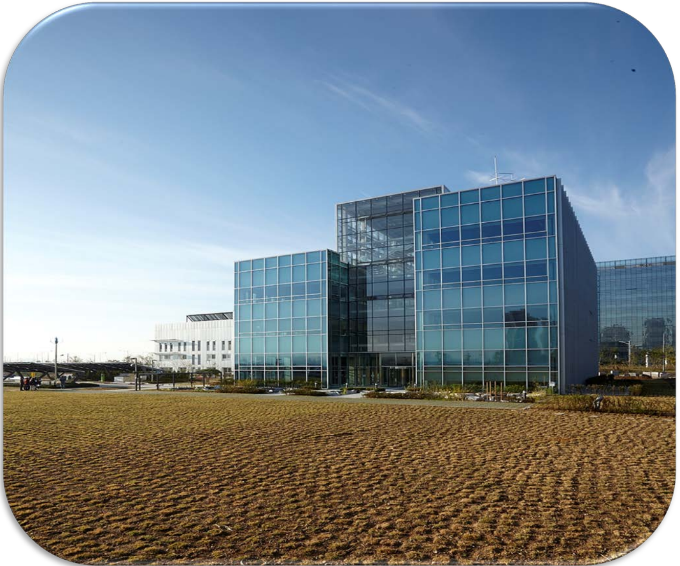
Posco Green Building in Yeosu, Republic of South Korea, features Uponor heating and cooling system with ceiling comfort panels
