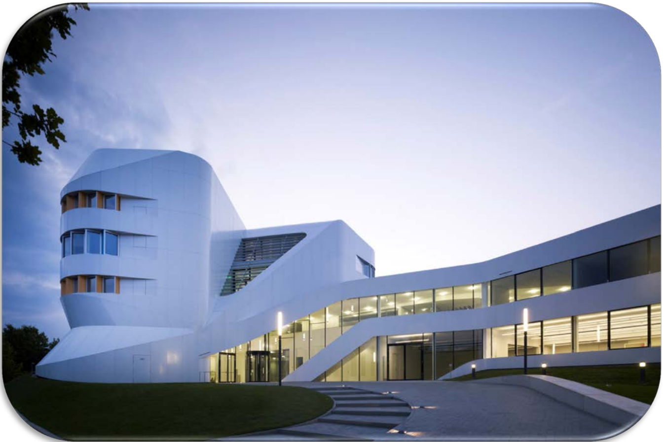
Geothermal energy solution, Centre for Virtual Engineering, Stuttgart, Germany
