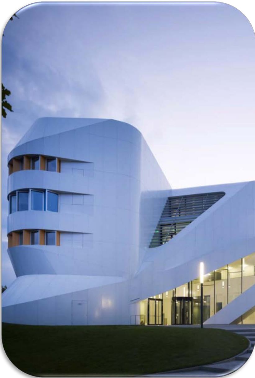
Geothermal energy solution Centre for Virtual Engineering, Stuttgart, Germany
