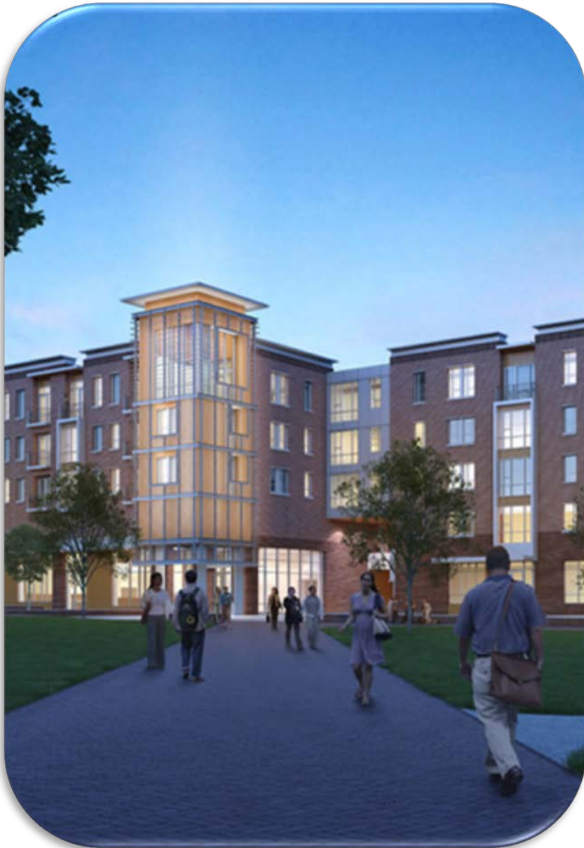
PEX plumbing at North Carolina State University housing, USA
