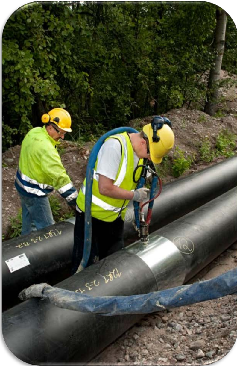
Installing pipes for district heating
